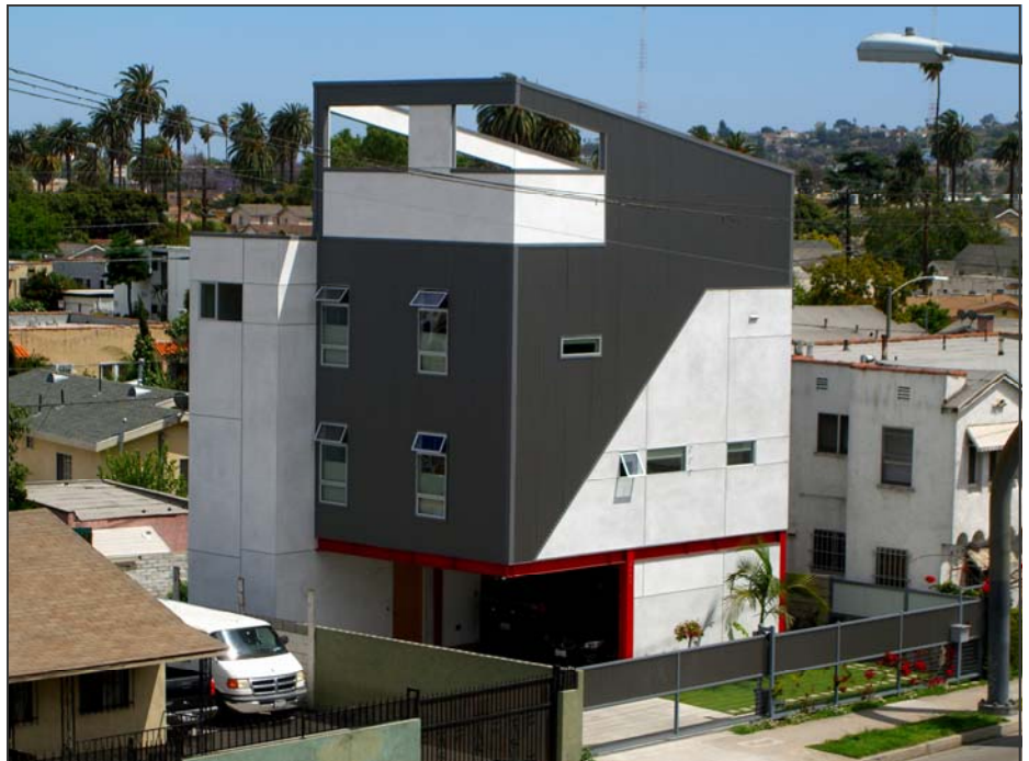
The 1,600-sq.-ft. home in Los Angeles designed and built by architect Jayna Cooper is a model of sustainability. It includes an energy-efficient, duct-free Daikin AC® 4-port Multi-Split system for heating and cooling.
